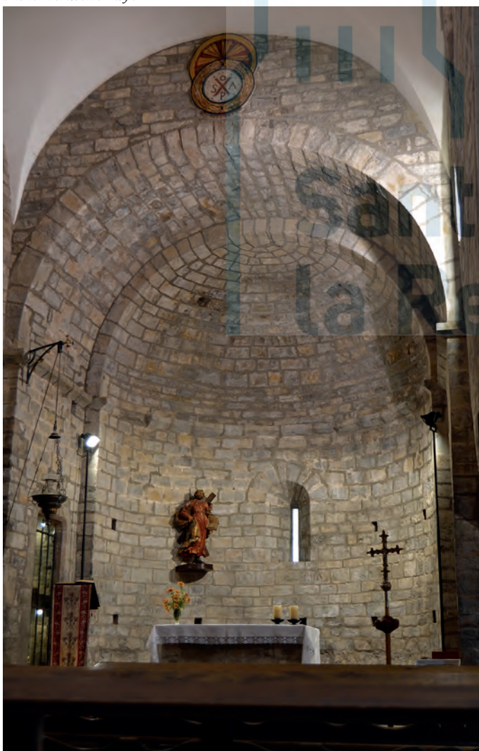
Interior del ábside mayor
