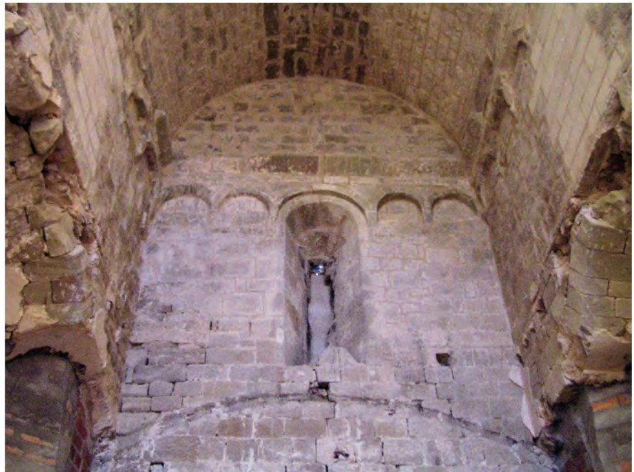
Interior de la capilla mayor
