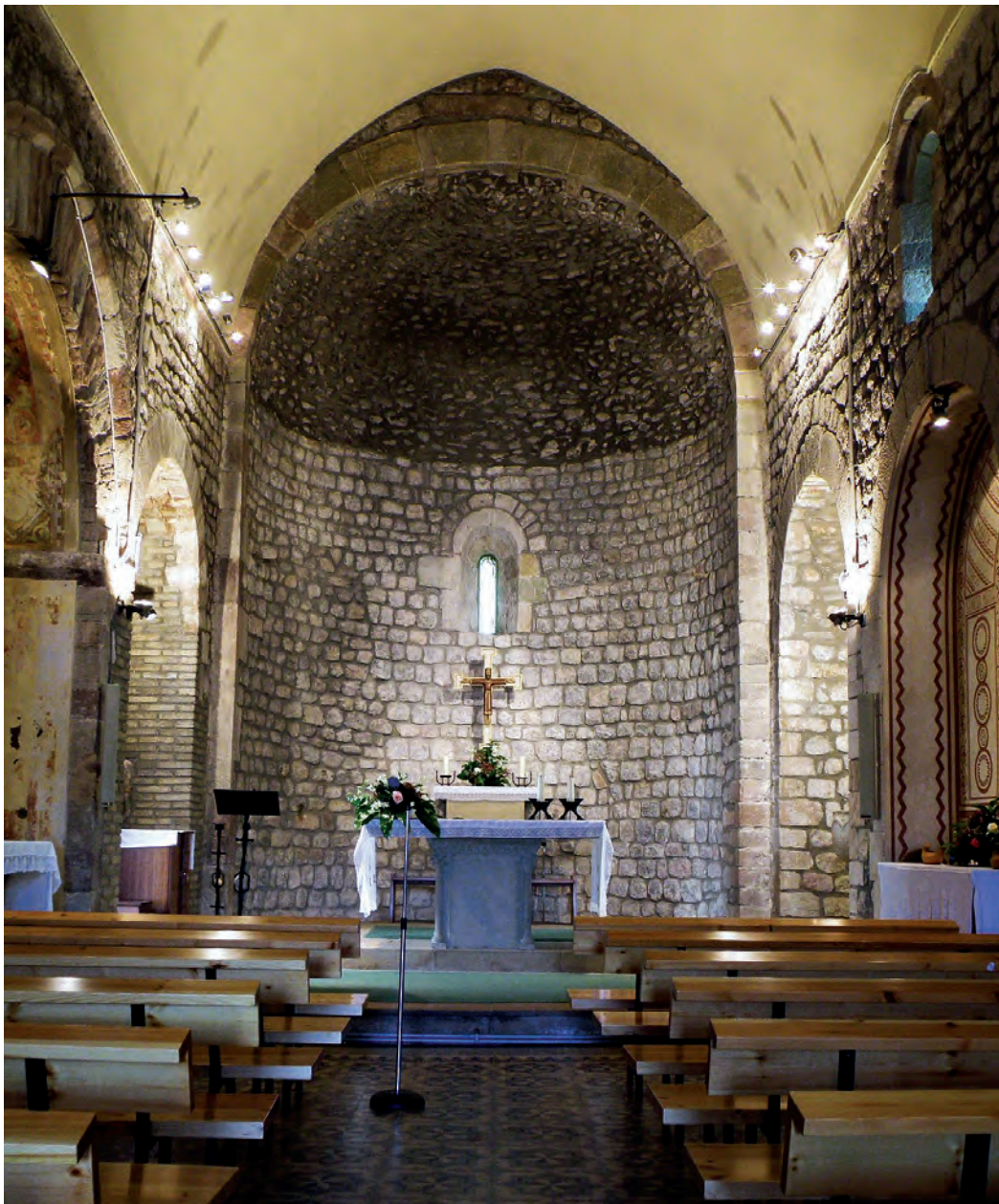
Vista general del interior
