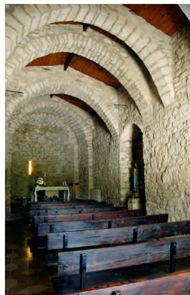
Vista general del interior
