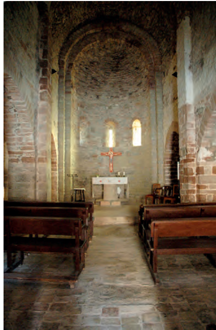
Vista general del interior
