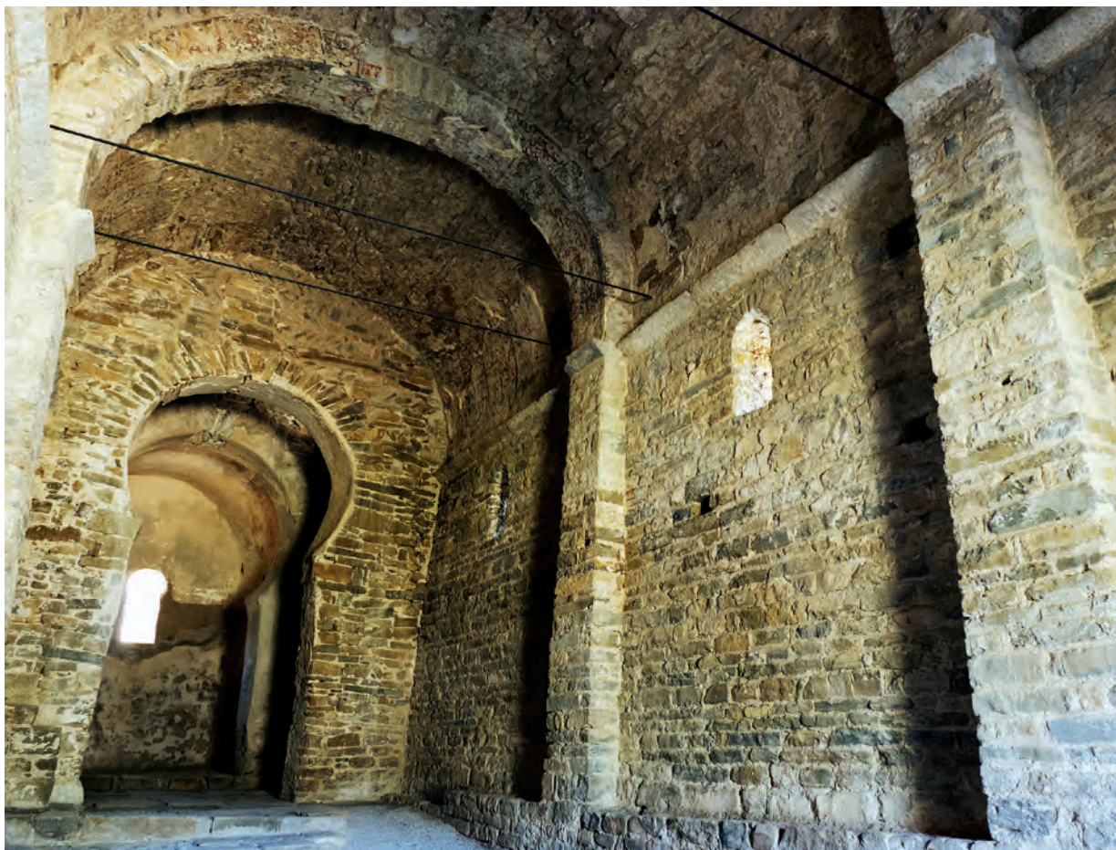
Vista general del interior
