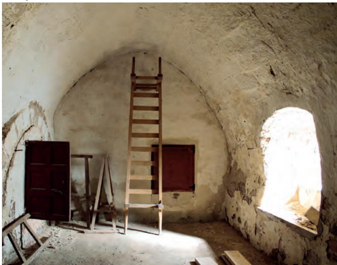
Vista general del interior
