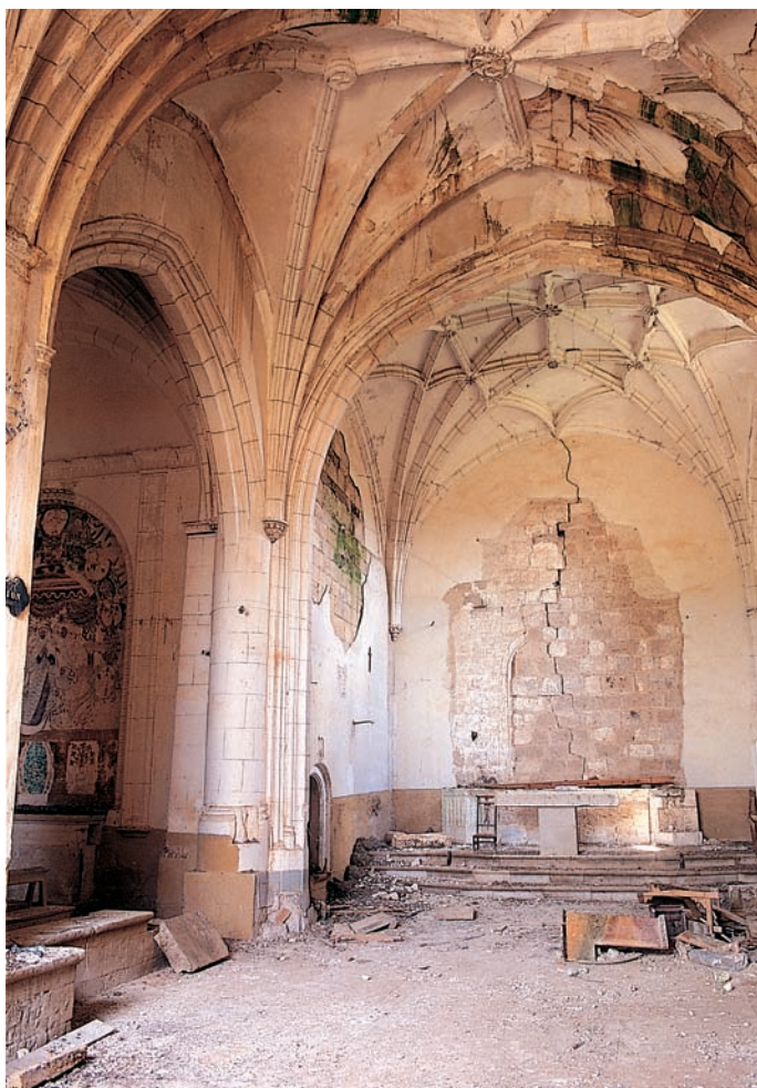
Vista general del interior
