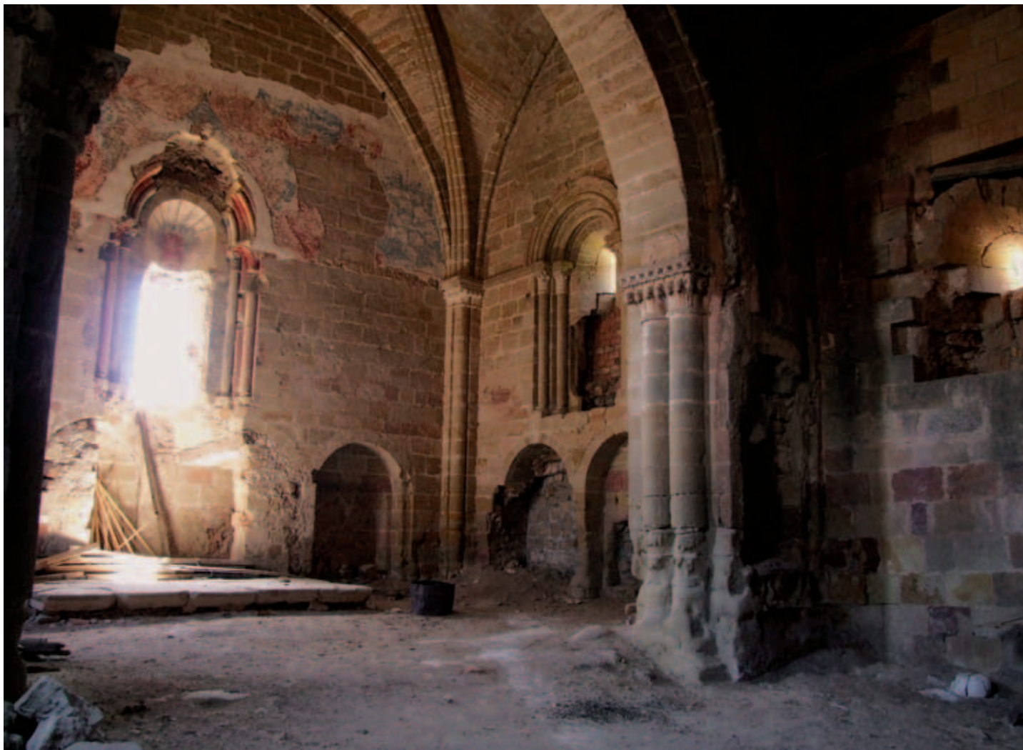
Interior de la capilla mayor
